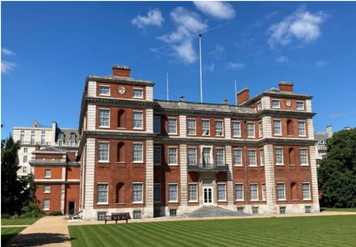
Marlborough House - the headquarters of the Commonwealth - on a summer's day
